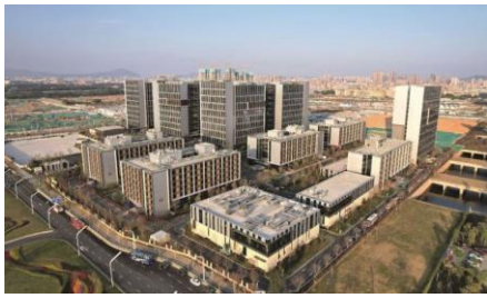
By robots, for robots ... the real Shenzhen Bay International Hotel, designed and built using XKool. Photograph: XKool
