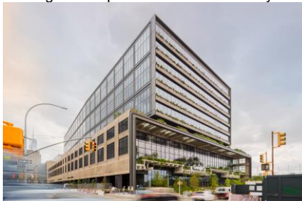
The building encompasses an adapted 1930s rail station, topped with nine additional floors
